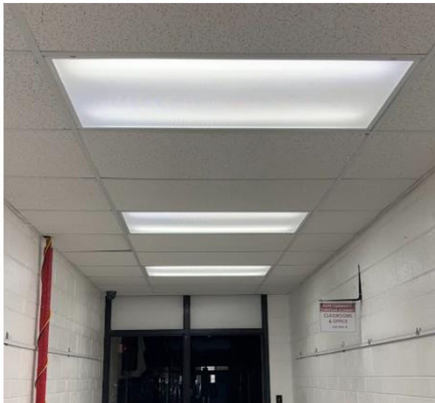
Typical Recessed Fluorescent Fixture
