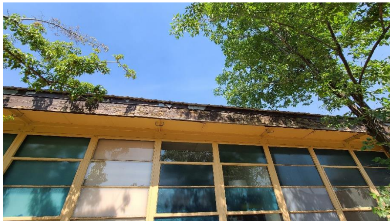
Peeling Paint and Rot on Wood Eaves
