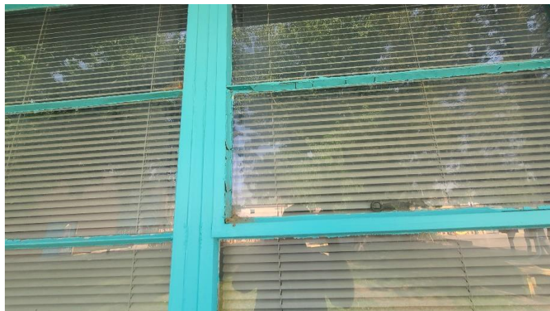
Deteriorated Glazing
