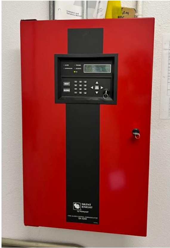
Fire Alarm Control Panel
