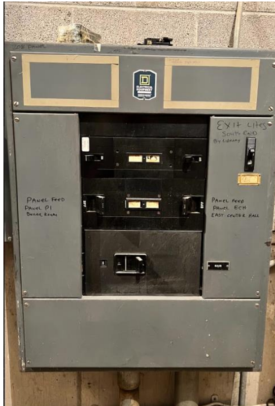
Figure 16: Existing 1-Phase Electrical Service MDP
