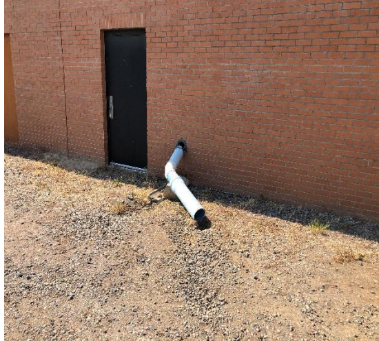
Roof spout drain on north side
