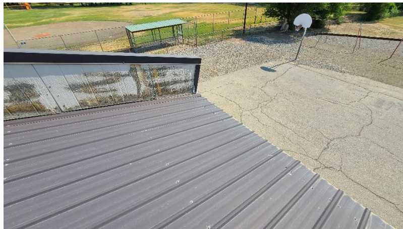
Lifted Fasteners on Roof
