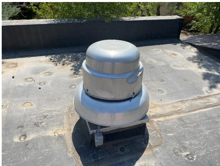
Bathroom Exhaust Fan on Roof
