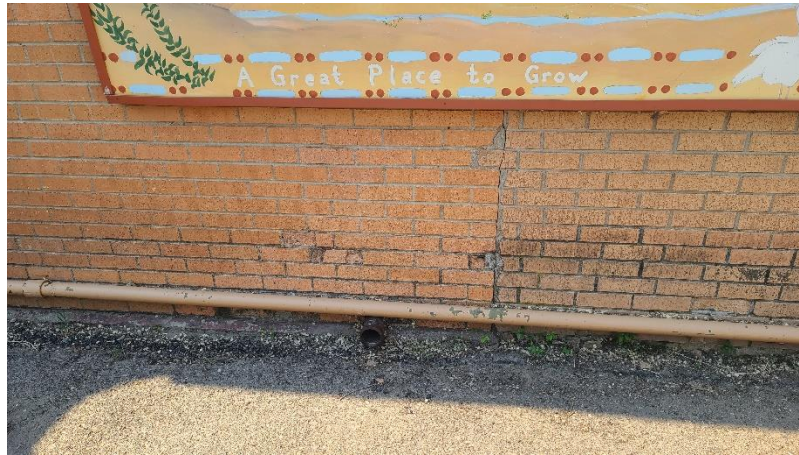
Spalled Brick and Missing Mortar
