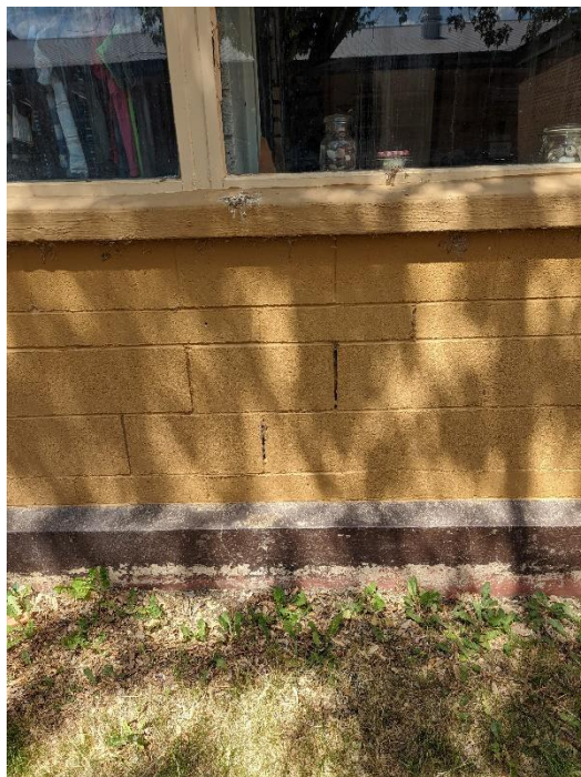
Masonry Cracking
