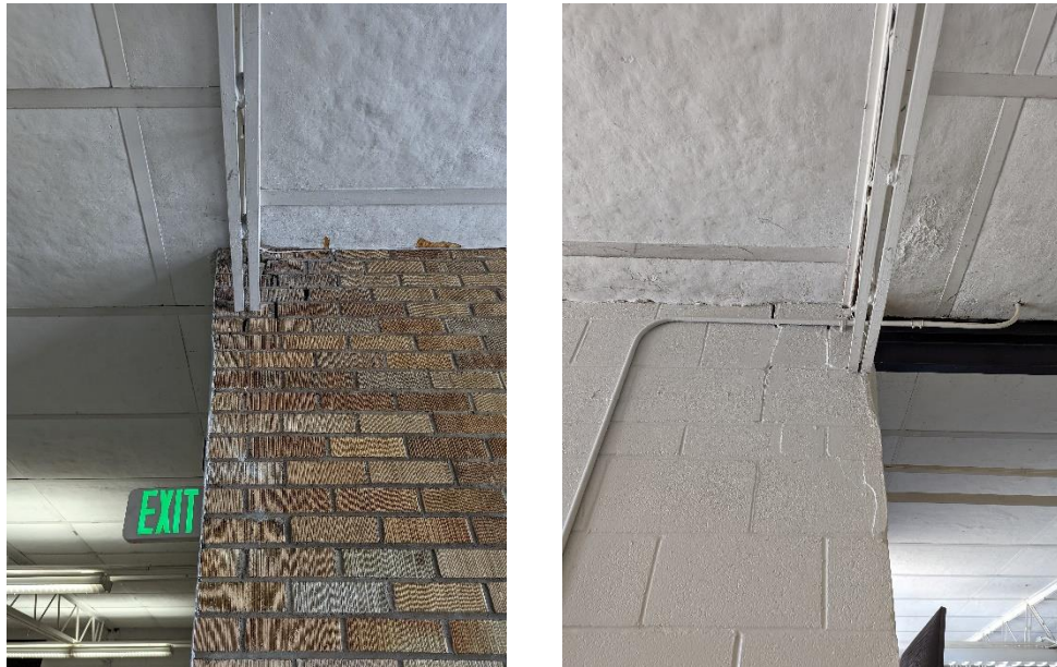
Compromised Joist Bearing
