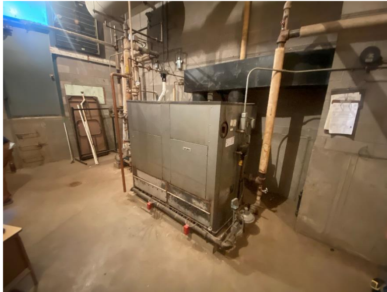
Existing Gas-Fired Furnace
