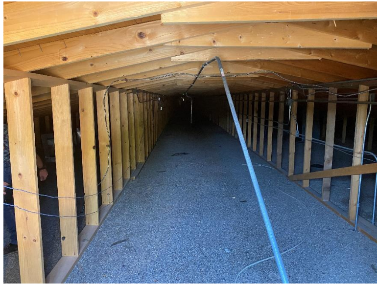
Typical Missing Fire Sprinklers in Attic Space
