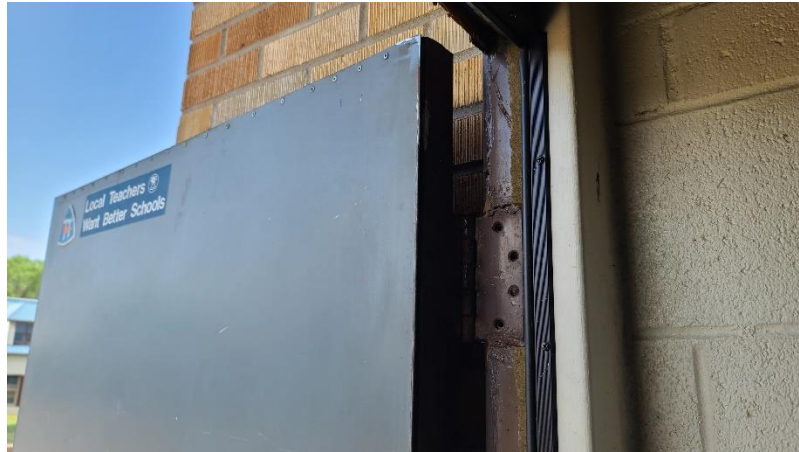
Corroded Exterior Door
