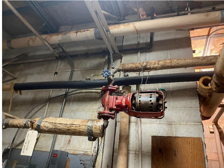
Damaged Hot Water Pipe Insulation
