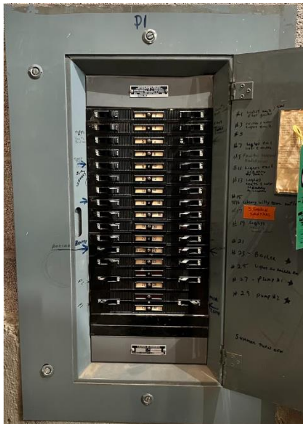
Typical 1-Phase Service Electrical Panel
