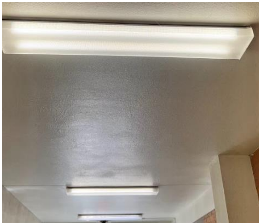
Typical Surface Fluorescent Fixture
