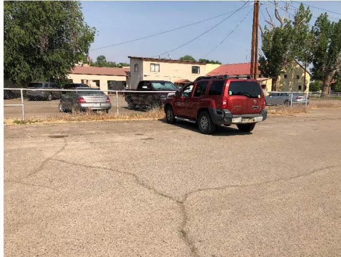
Paved parking area no west side with cracking.
