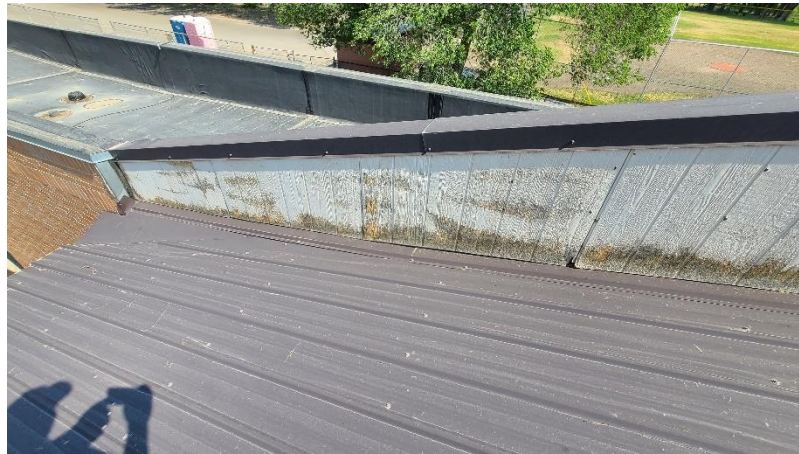
Mildew and Water Damage at Parapet Wood Siding
