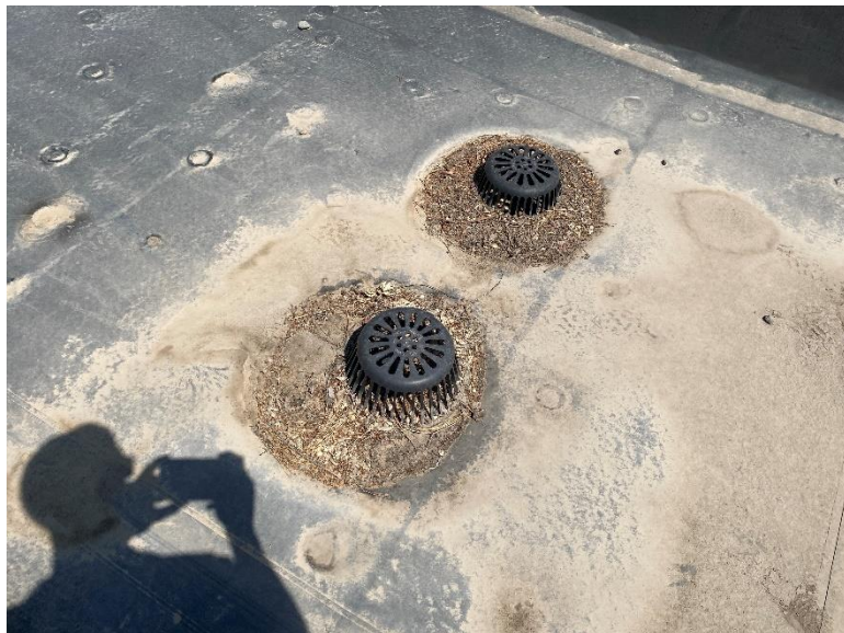
Clogged Roof Drain
