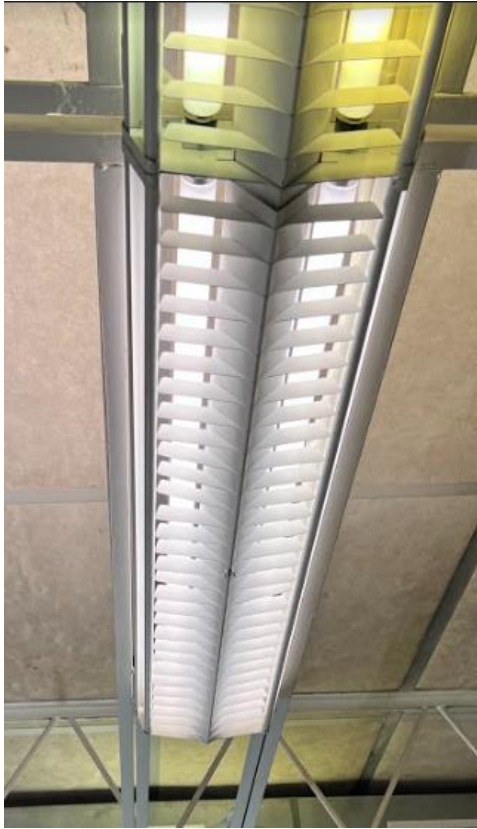
Typical Suspended Fluorescent Fixture
