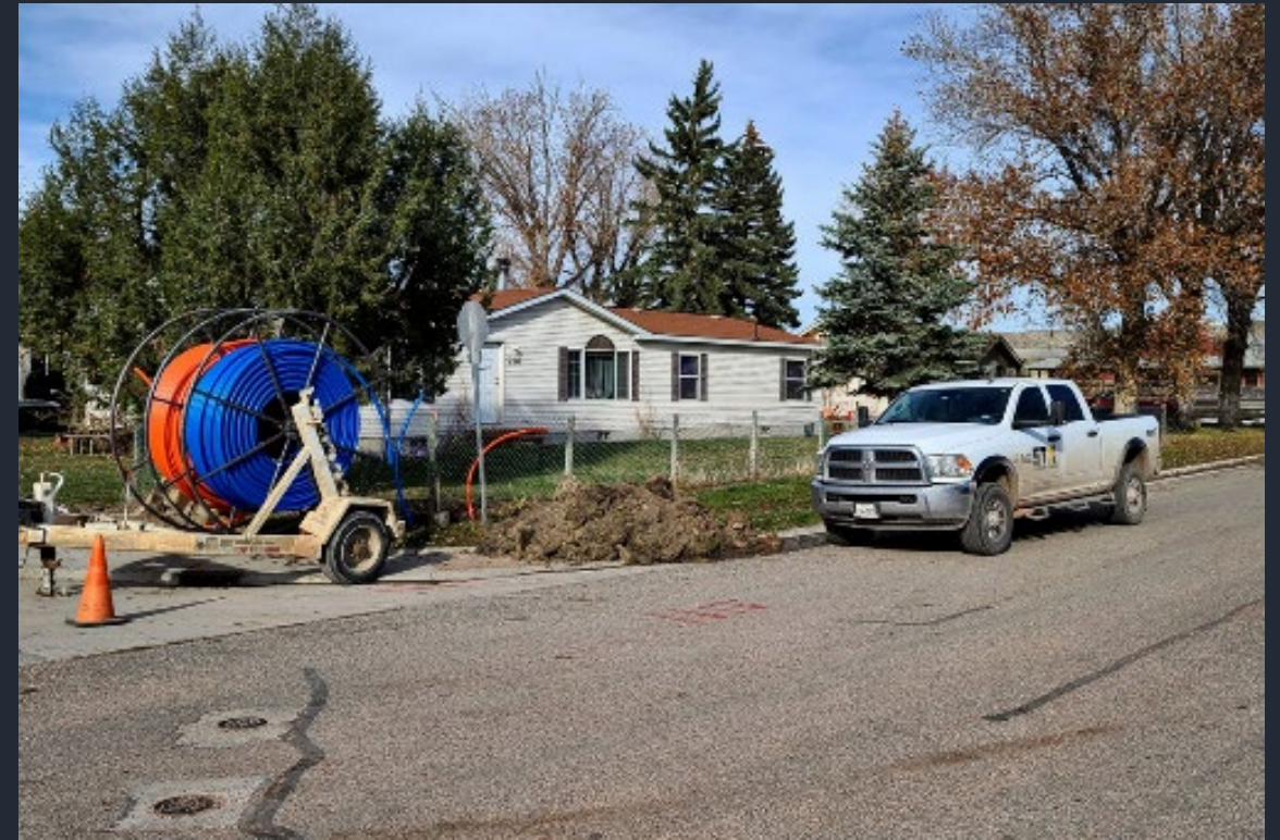
Bore Pit at end of bore hole
